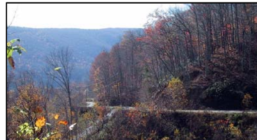
Mountain-hugging road segments
